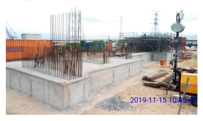
Eastern Approach - Casting station - Installation of reinforcement for pile cap
