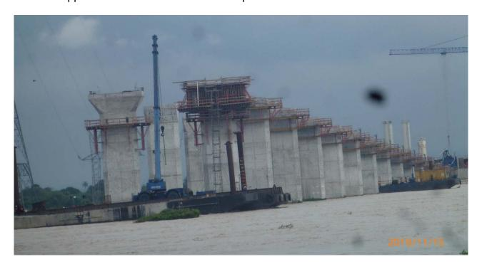
Niger Bridge Axis 260 - Pier table - Bottom part (North and South) completed
